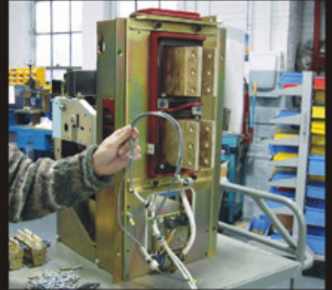
Removal of sensor cable(s), completely from circuit breaker.
