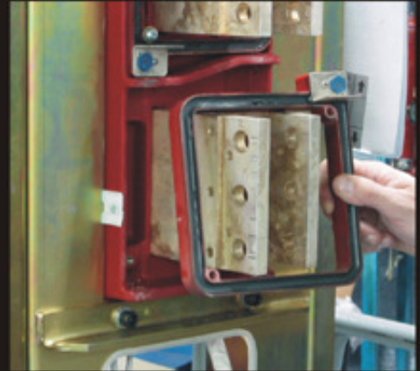
Remove old sensor completely from breaker bus. Repeat for each.
