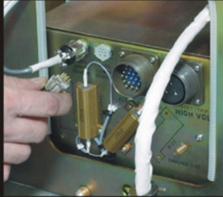
Remove first sensor cable from trip unit.
