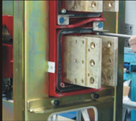
Remove second of two phillips screws from old sensor.
