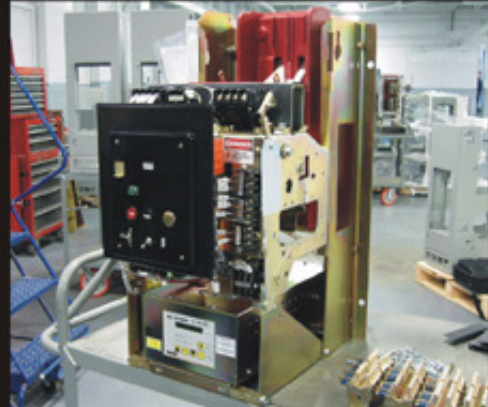
FBK circuit breaker with CP trip unit after replacement. Front View.
