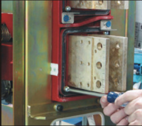
Remove first of two phillips screws from old sensor.
